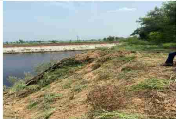
Photo 5: Lagoon-3 being dismantled
