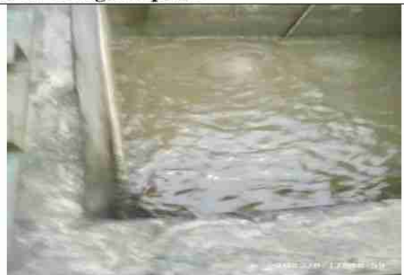
Photo 16: ETP inlet collection tank in bottling plant
