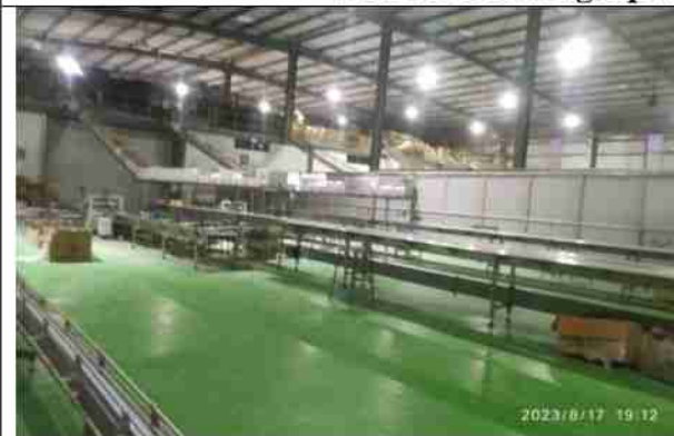
Photo 15: Bottling plant of unit
